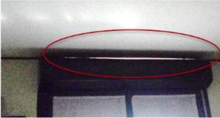
Draughts of cold air through air gaps between windows frame and slab/wall
